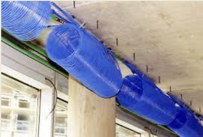
Fitting coils to slab
