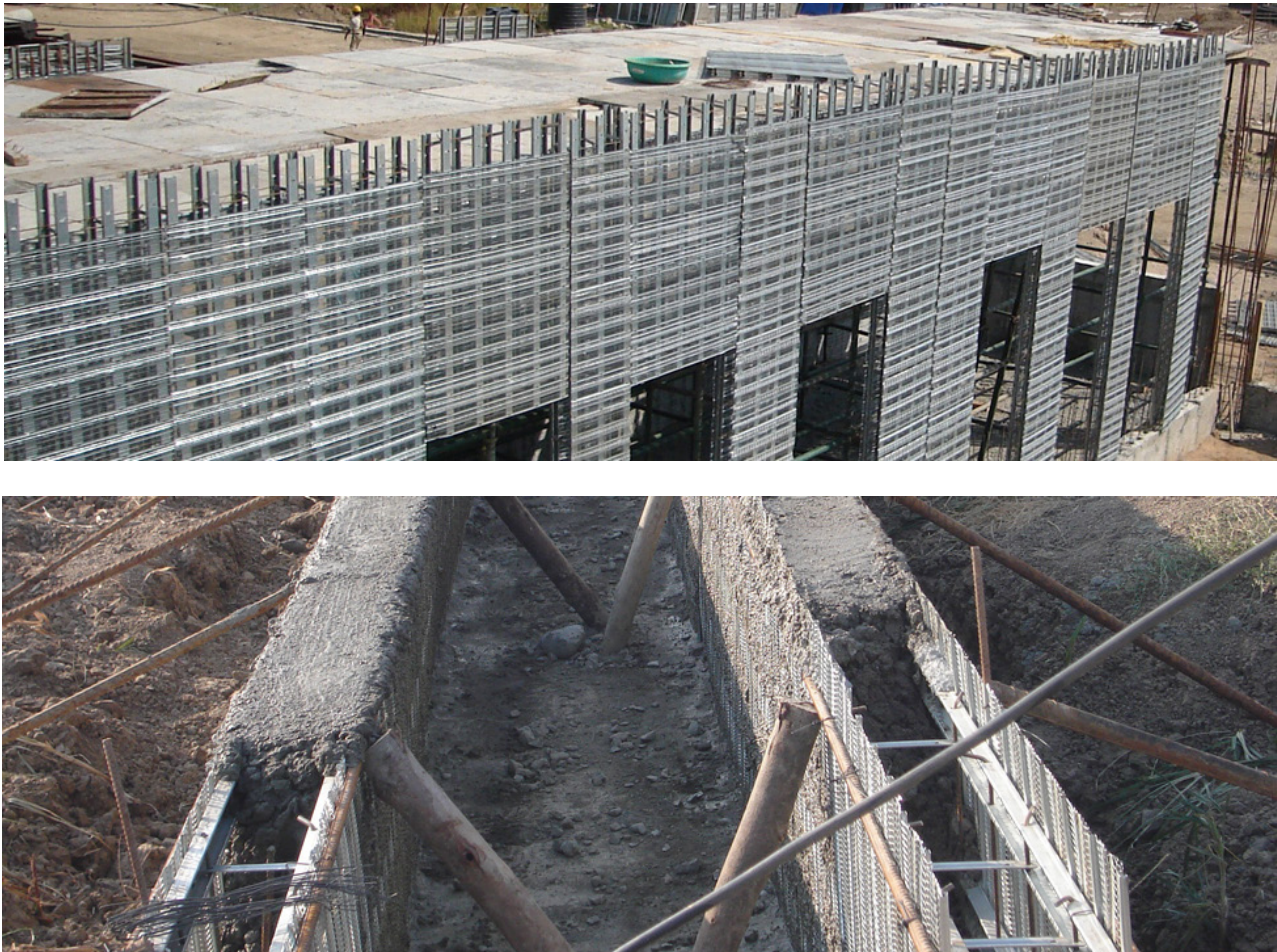
Figure 26: Photographs of the assembly of 'Coffor' panels without insulation (first) and filled with concrete on-site (second). Source: (Coffor Construction Company LLD, n.d.)
