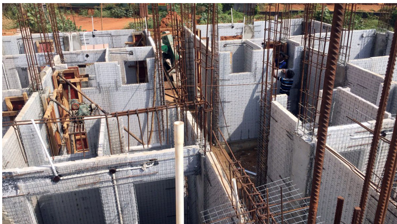
Figure 18: Photograph of an affordable housing construction employing Reinforced EPS core panels Source: (BMTPC, 2017)
