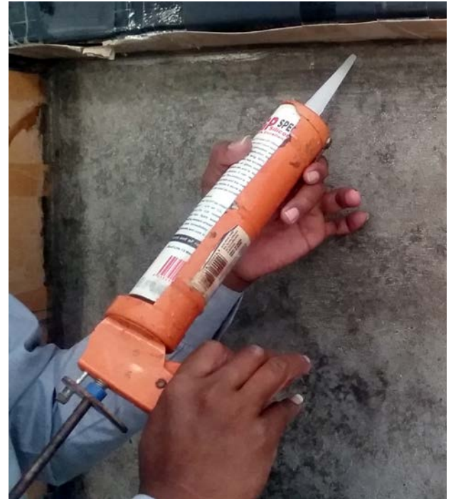
Figure 8: Photographs showing sealing procedure with XPS (left) and silicone sealant (right) to avoid heat transfer through gaps
