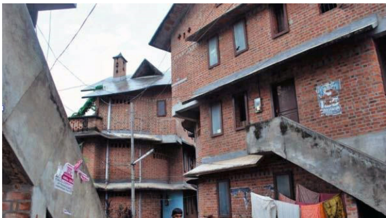
Figure 10: Photograph of a housing project by Laurie Baker employing rat-trap bond wall assembly Source: (Saurabh, 2015)
