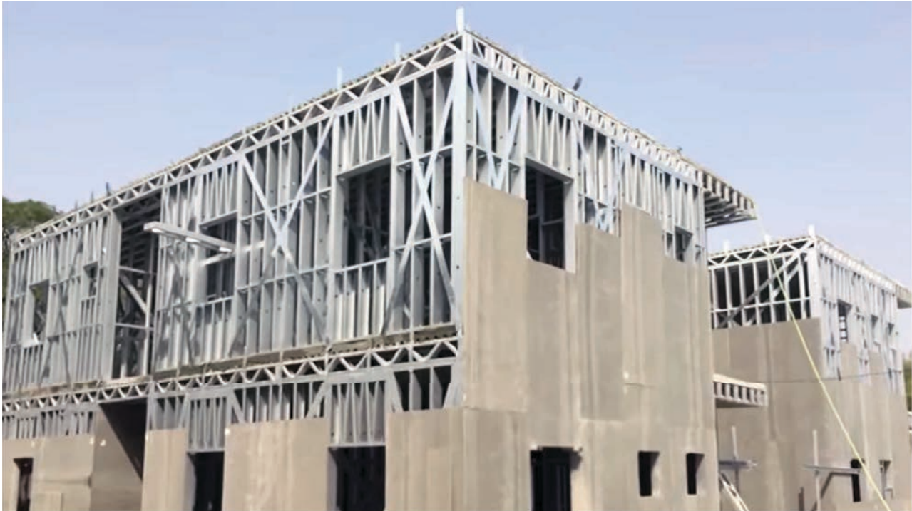
Figure 13: Photograph showing walls and floor plates of LGFSS assembled at a site. Source: (BMTPC, 2018b)
