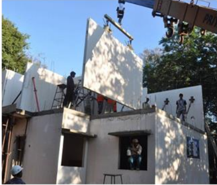
Glass fibre reinforced Gypsum Panel (GFRG)
