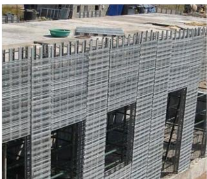
Structural stay-in-place coffer formwork system
