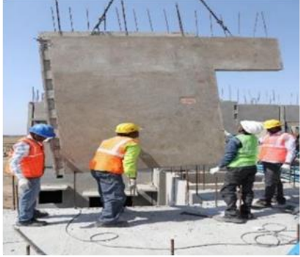
Precast construction technology
