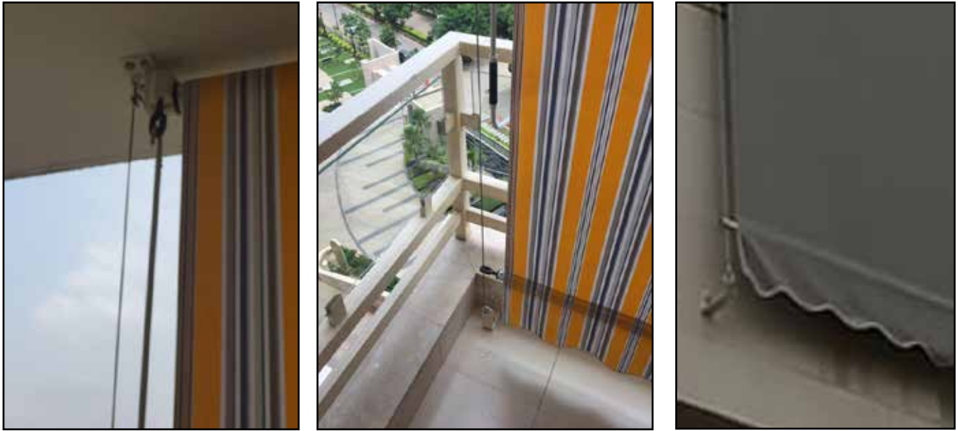
Fig. 3d: Cable-guided Installation
