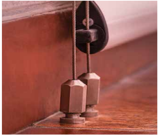
Fig. 2.1.1b: Cable Anchored to Floor
