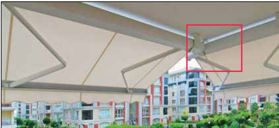
Fig. 3c: Awning Anchored with Ceiling Brackets
