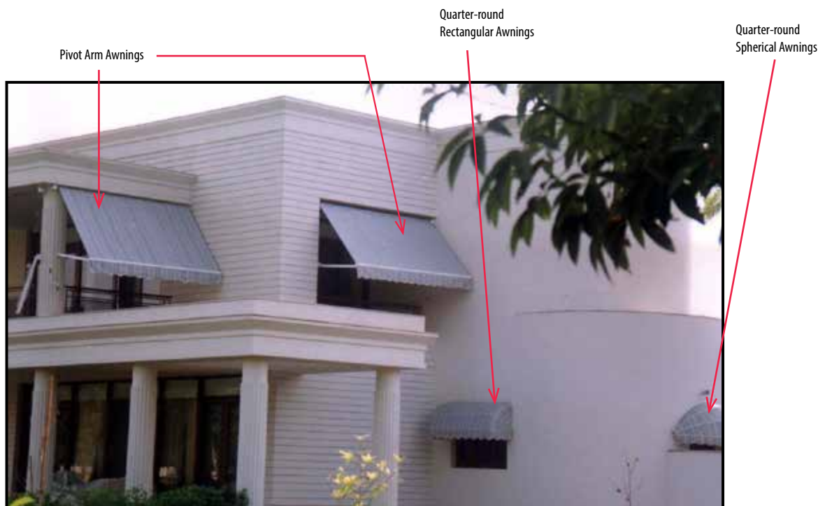
Fig. 5.2: Pivot Arm, Quarter-round Fold (Spherical and Rectangular) Awnings: Private Residence, New Delhi
