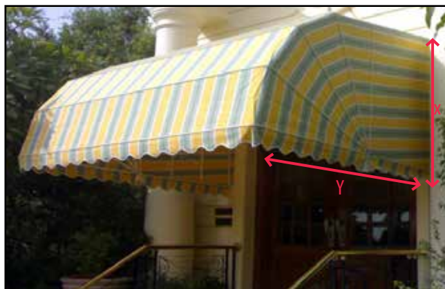
Fig. 4.3b Perspective View of Quarter-Round Foldable, Rectangular Awning
