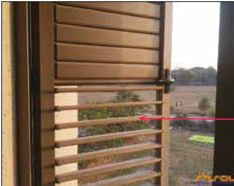
Fig. 5: Shutter with Adjustable Combination Louver Window in a Private Residence at Ahmedabad
