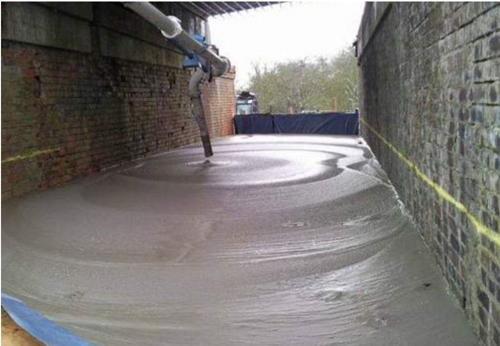
Figure 5: Foam concrete installation on roof
