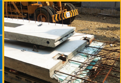
A Picture of pre fabricated sandwich panels
