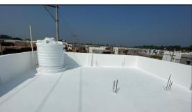
It can also have other features such as infrared-reflective pigments, which further enhance its ability to reflect heat. In addition, they also protect the roof surface from chemical and water
