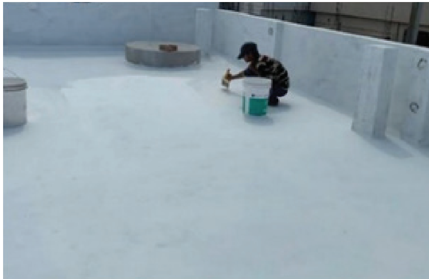
Figure 2. Five layers of coatings were applied on roof of selected houses.
